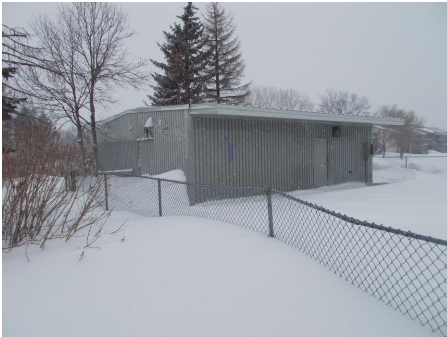
PHOTOGRAPH 5: Showing the exterior of the Wading Pool building.
